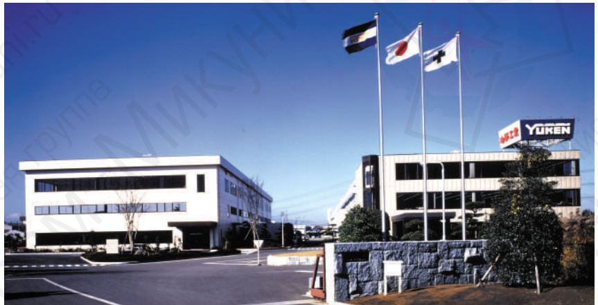
● Sagami Plant Front Gate
